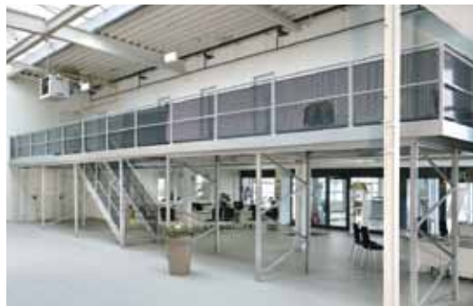
This META steel platform provides space for employees in 8 office rooms
