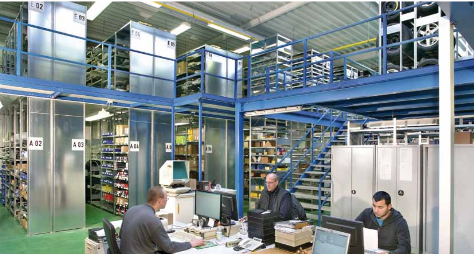
An open-plan warehouse with two-tier META QUICK® system is optimised to meet customer requirements, and all roads lead to the service points
