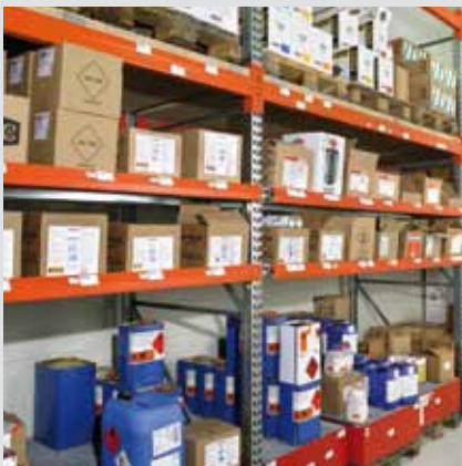
The explosion-protected hazardous goods store holds items identified by the hazardous goods pictogram
